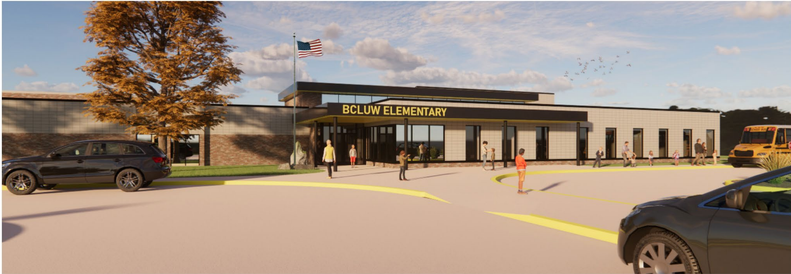
Elementary Main Entrance and Addition
